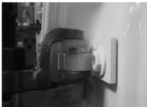
Figure 7. Gap between Door and Locking Nut
